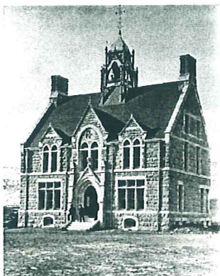
Cutler Hall was built to house classrooms, a library, an auditorium/chapel and administrative offices in 1880. Peabody and Stearns, Boston, architects (photo c. 1880).
