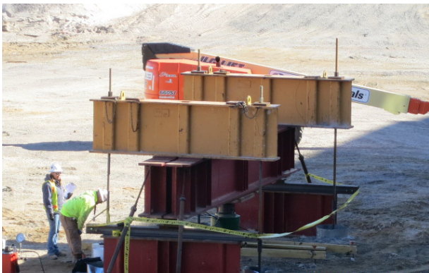
(Top) Adair Stevenson watching a Partial Displacement Pile Load test.
